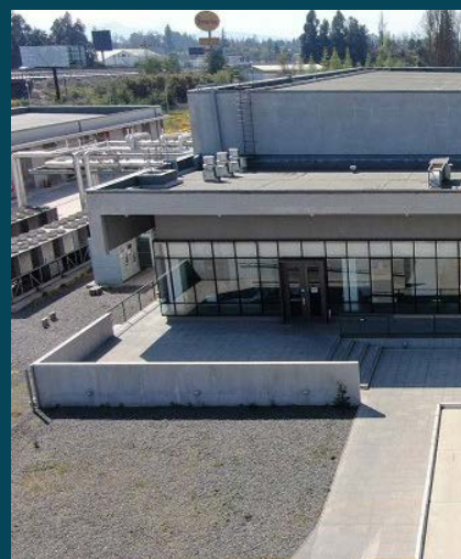
Data Center Paine
