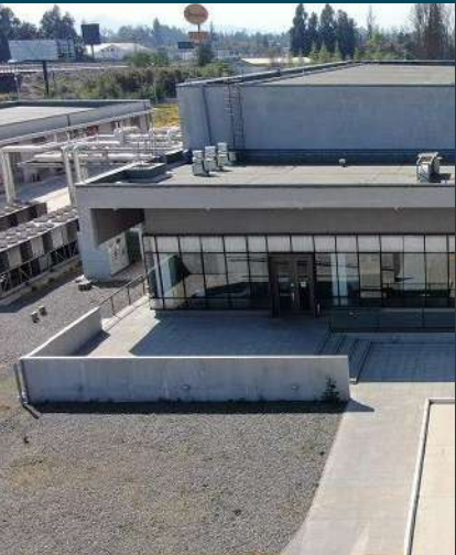
Data Center Paine
