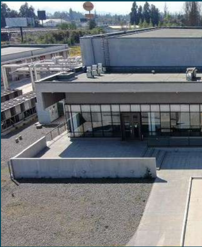
Data Center Paine
